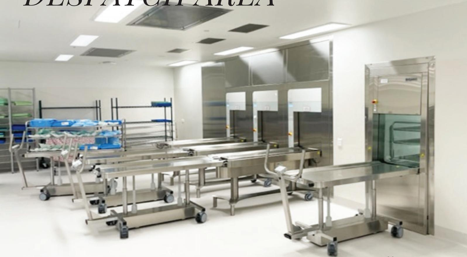
All sterilisers are pass-through and equipped with auto unloaders. There is sufficient room for keeping clean case carts and shelving is provided for keeping sterile stock for wards and other facilities. Once the sterile RMDs are ready to be delivered, they are loaded on to the case carts with supporting transport trays and deliver to destinations by SSU staff.
