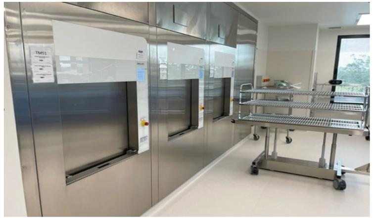
Two low temperature sterilisers and three steam sterilisers are in operation now and there is a provision for the fourth steam steriliser as future proof. Heat sealers, Insulation tester, Dental oiler, Air blower with cabinet are also provided.
