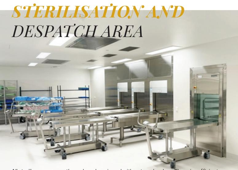
All sterilisers are pass-through and equipped with auto unloaders. There is sufficient room for keeping clean case carts and shelving is provided for keeping sterile stock for wards and other facilities. Once the sterile RMDs are ready to be delivered, they are loaded on to the case carts with supporting transport trays and deliver to destinations by SSU staff.
