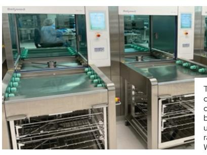
There are 4 batch washers and one cart washer and a pass through drying cabinet in the department. All the batch washers have auto loading and unloading conveyers and automated rack return device also provided. Washing sinks and eye wash facilities are also provided for the staff.
