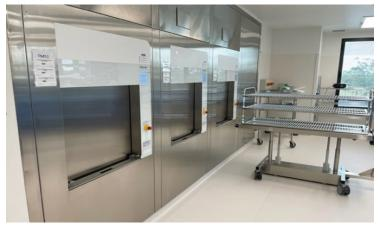
Two low temperature sterilisers and three steam sterilisers are in operation now and there is a provision for the fourth steam steriliser as future proof. Heat sealers, Insulation tester, Dental oiler, Air blower with cabinet are also provided.
